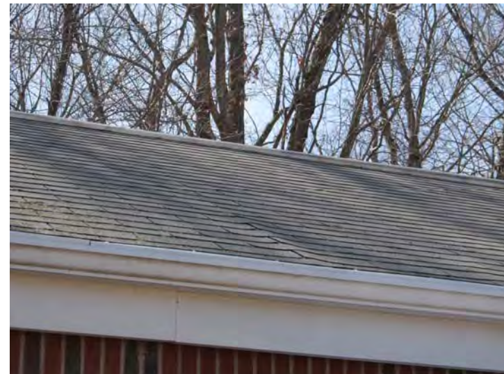
Roof shingles in fair condition – Isolated areas of warped/buckled roof sheathing noted
