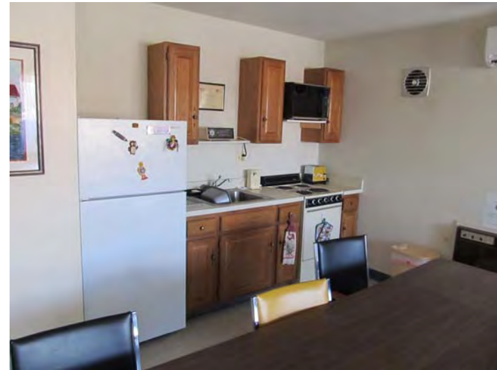
Kitchen area located at one end of community room – Note lack of knee clearance space at sink and work surface
