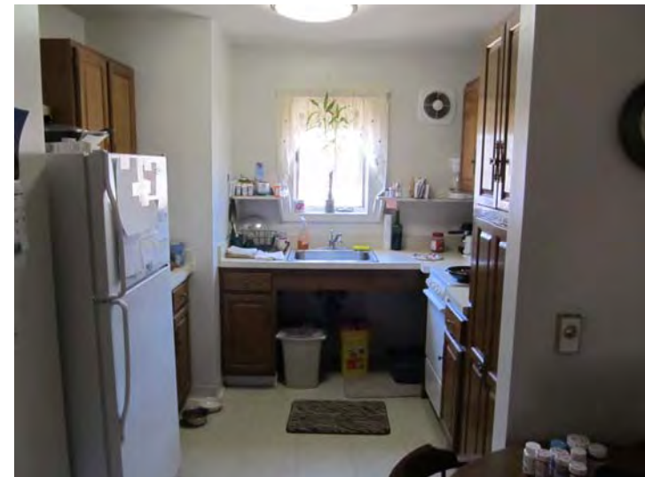
Typical handicap accessible unit kitchen – Note lack of a thirty-inch wide work surface with necessary knee clearance space
