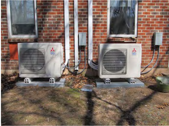
Typical exterior condensers for heat pump systems that were recently installed at all units
