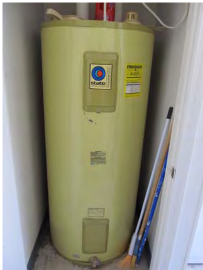
Electric domestic hot water tank serving community building – Serviceable but beyond end of expected useful service life
